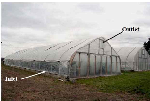
Figure 4. Natural Ventilation – Inlets and Outlets
