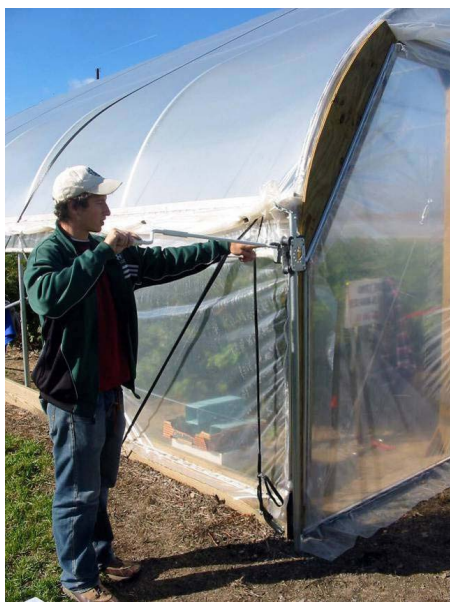
Figure 9. Manual roll up of sidewalls
