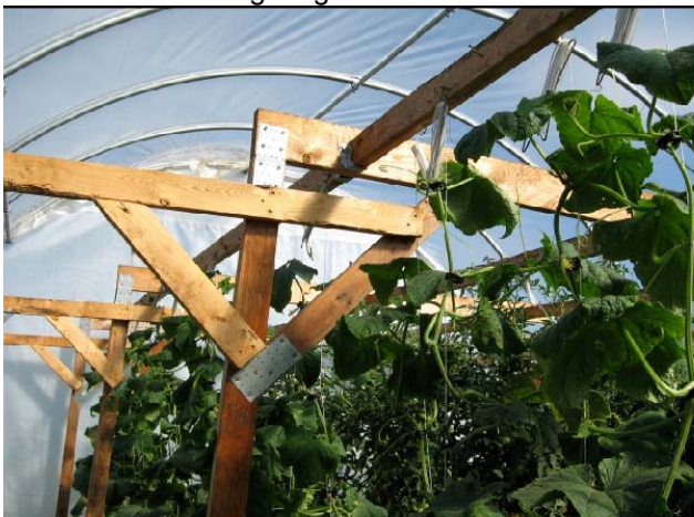
Figure 11. Optional extension adds an additional row to each side of mainframe
