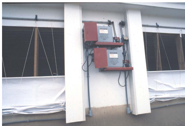
Figure 10. Automated temperature sensor and inlet controller
