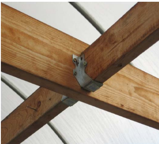
Figure 7. Joist U hanger using square headed screws for easy removal in fall. Mark 2X4 if you use a pin system so that stringer is used in same spot
