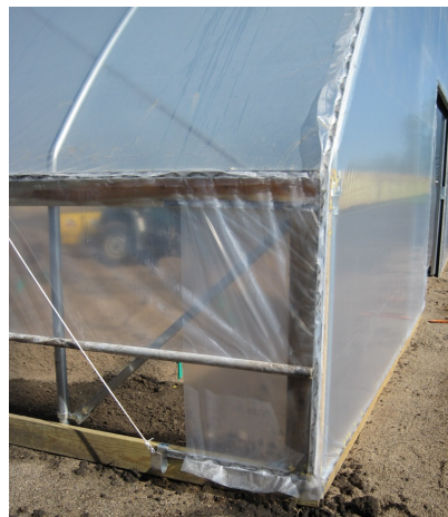
Figure 2. Plastic corner attached, Lamberton, MN (K. Bellina, University of Minnesota)
