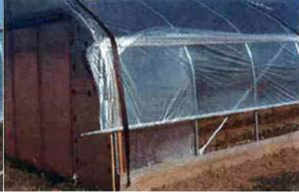
Figure 12. After plastic was attached
